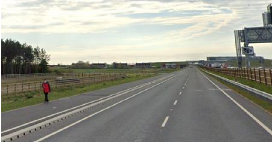
Local Access road NMU facility
